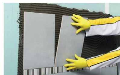
Tile onto Building Board
